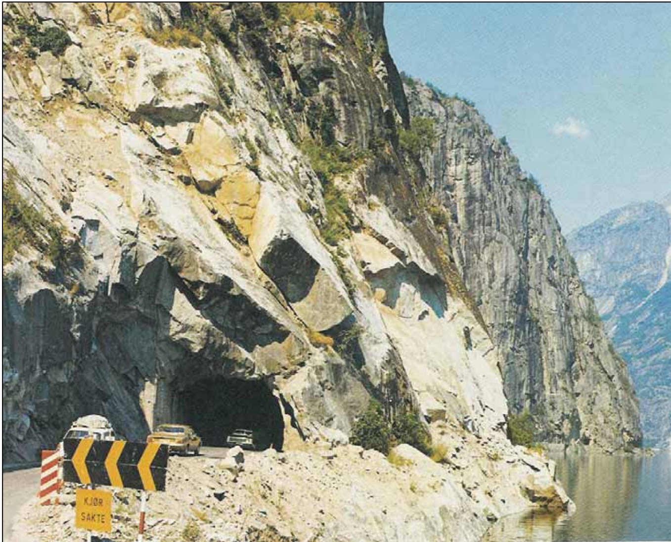
Near-surface example of high tangential stresses. NB'71
