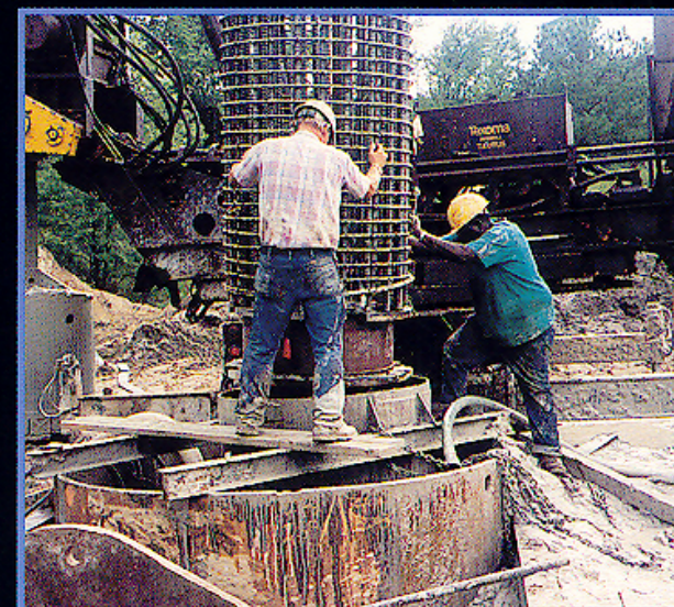
Installation of Osterberg cell into test shaft.
