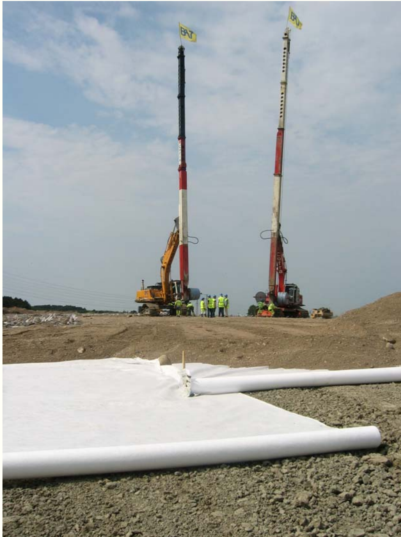
Drain Installation in Uppsala, Sweden
