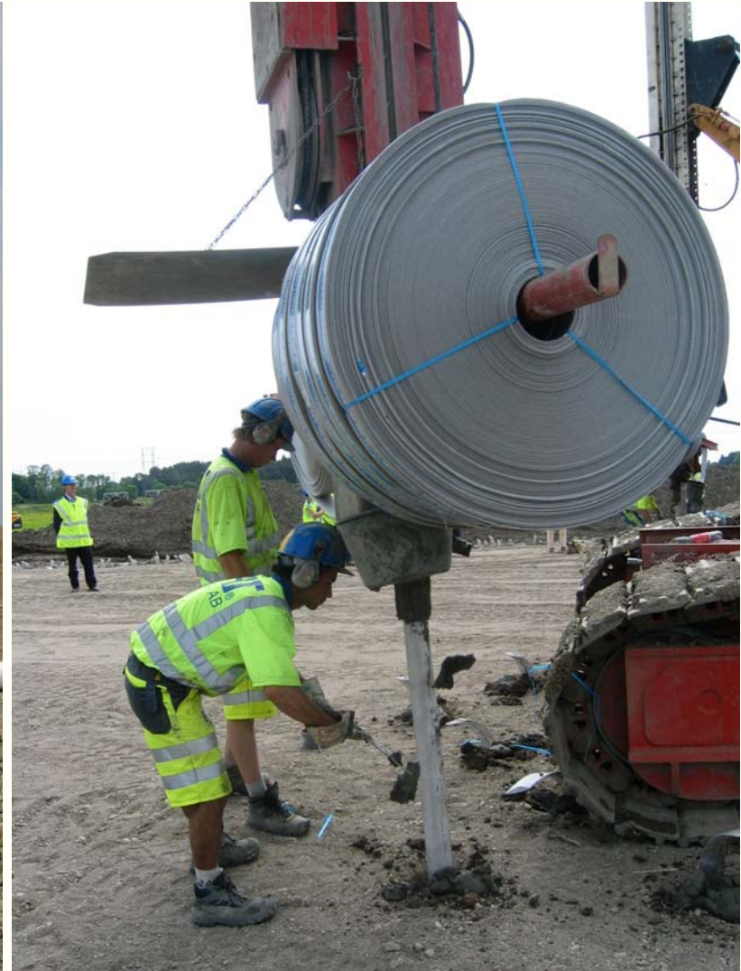
Drain Installation in Uppsala, Sweden
