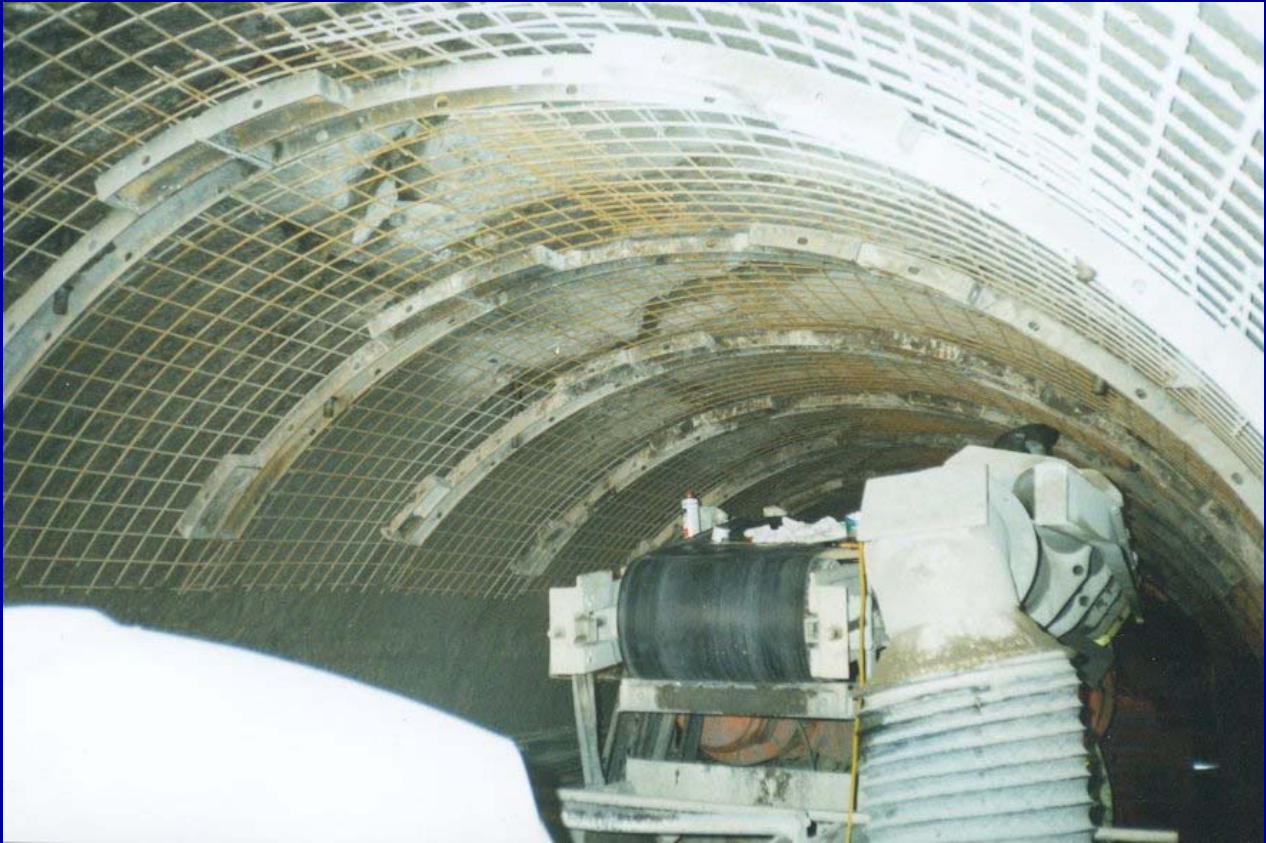
Typical support system behind the cutter head (liner plates, steel mesh, bolting)
