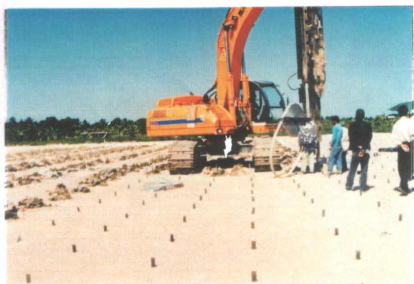
Fig. A-19 PVD Installation in Field
