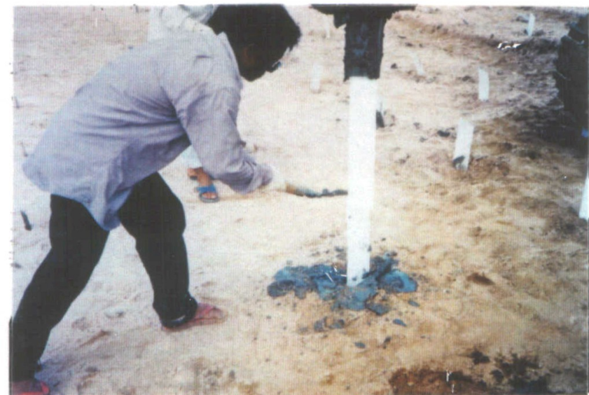
Fig. A-20 PVD Installation in Field
