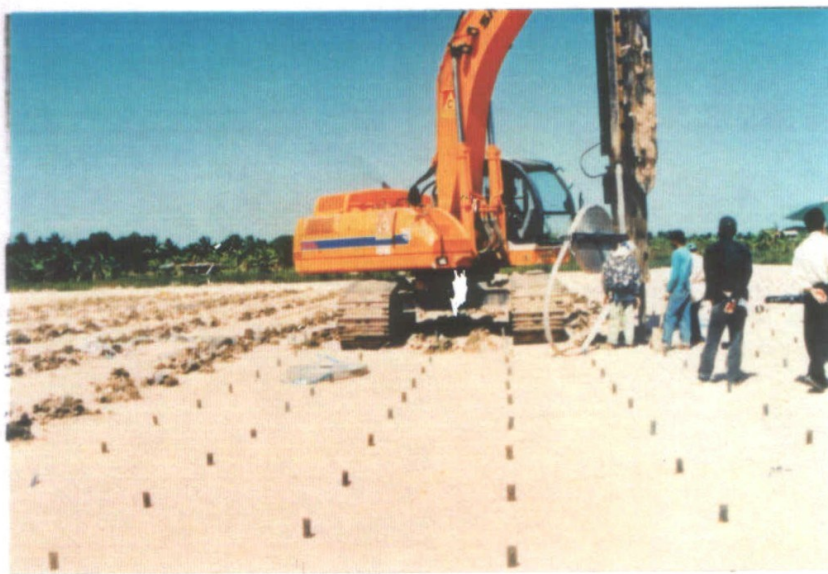
Fig. A-19 PVD Installation in Field
