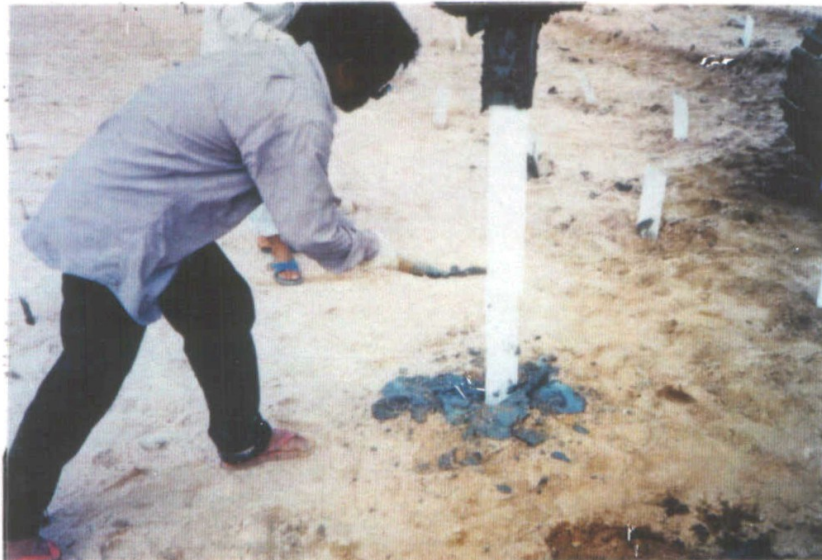
Fig. A-20 PVD Installation in Field
