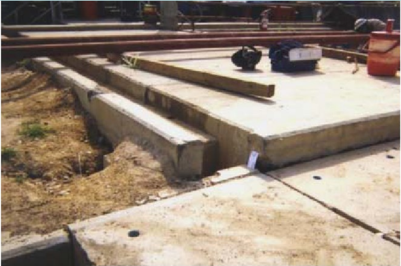
Differential settlement between piled and non-piled areas on non-treatment plant area
