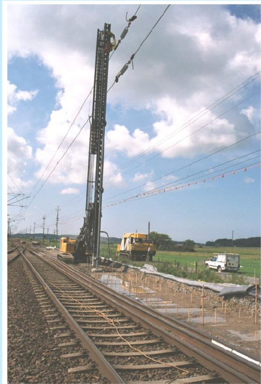
Figure 1. Deep mixing installation to reduce vibrations at high speed trains (Holm et al, 2002)
