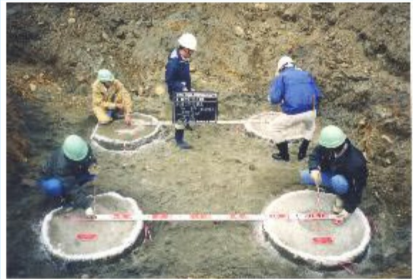
Figure 7.7 Mixed column with Dry mixing
