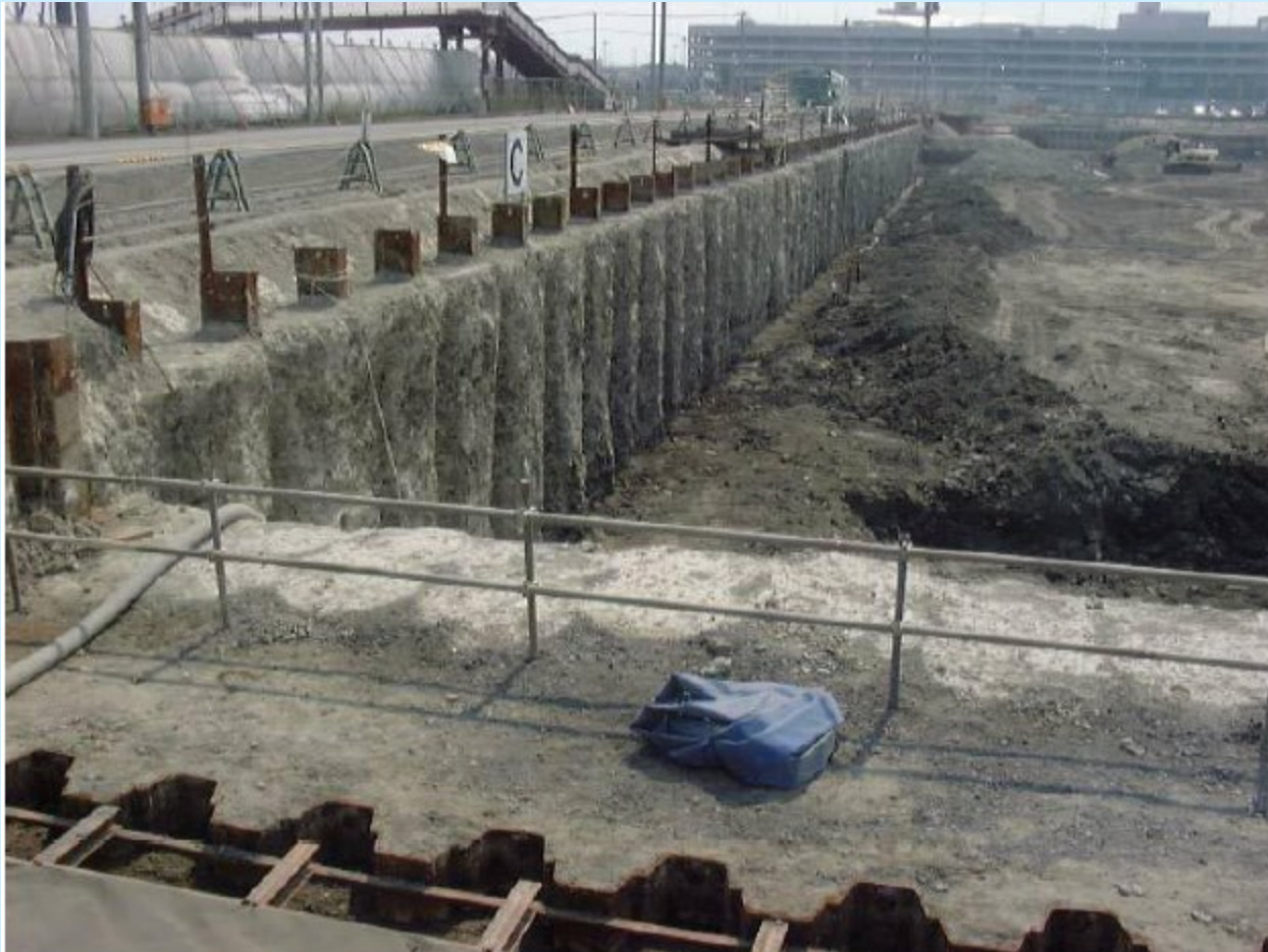
Figure 6.11 Photograph of Self-standing retaining wall in Haneda airport
