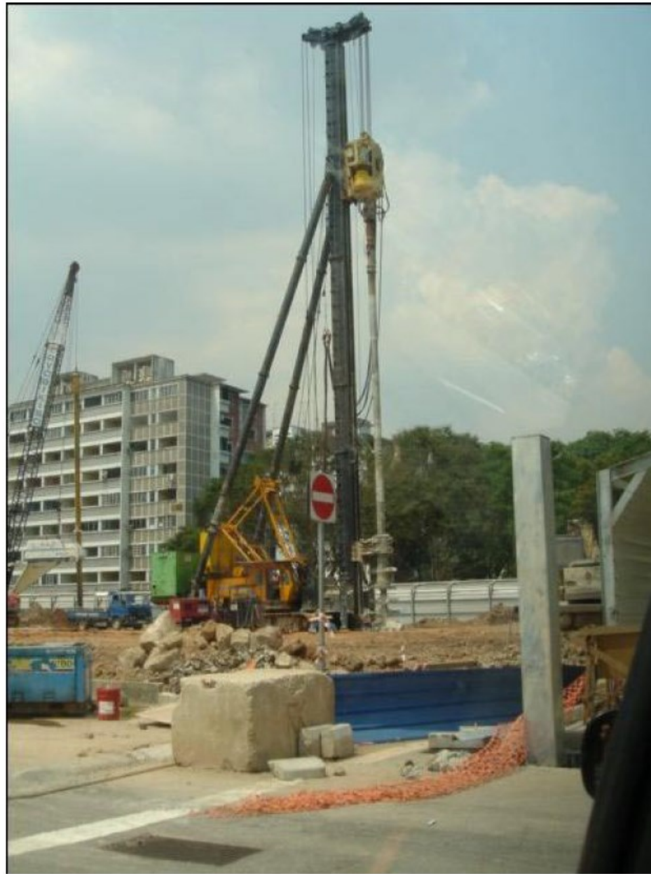
Figure 6.13 are the photograph of DMM machine for Self-standing retaining wall in Singapore
