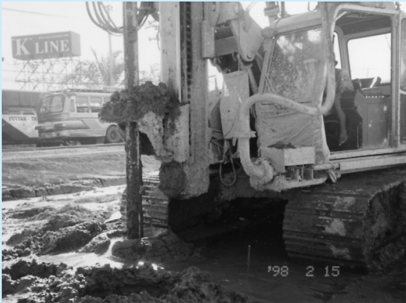
Fig. 6. (b) installation of cement piles by DMM machine
