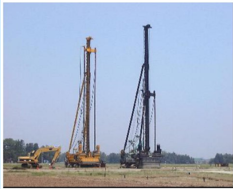
Figure 7.3 Dry type machine for two rods type
