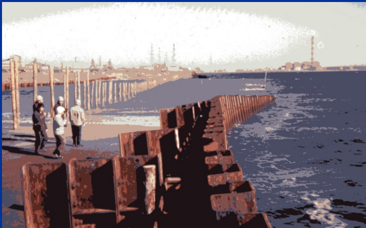
Failure of sea wall during backfilling
