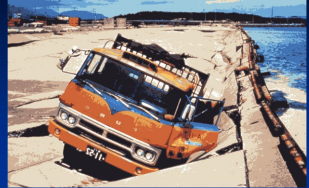
Liquefaction induced settlement of loose saturated sand
