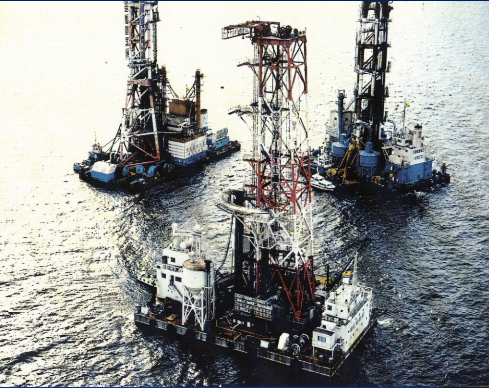
DMM barges working at TTB project site
