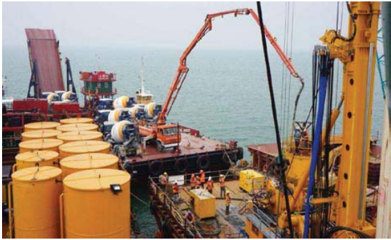
Figure 57. Concreting of Bored Pile
