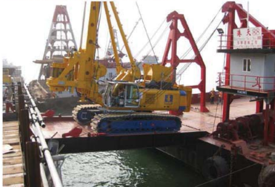
Figure 42. Actual Moving of BG 40 to Piling Platform
