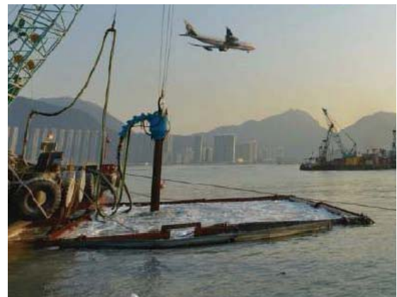
Figure 6. Stone Column Installation within Silt Curtain
