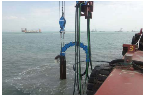
Figure 10. Work installation for Marine Stone Column in Low Headroom Condition
