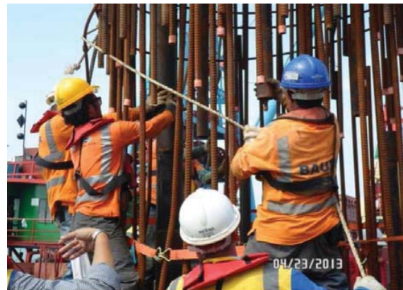
Figure 56. Rebar Cage Installation with Sonic Pipes
