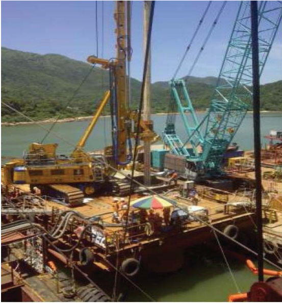
Figure 51. BG 40 Drilling on Platform
