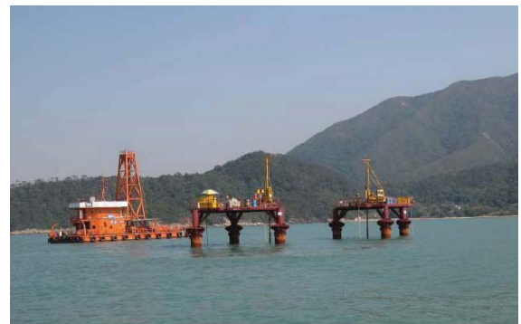
Figure 30. Soil Investigation at each Pile Location from Platforms or Barges
