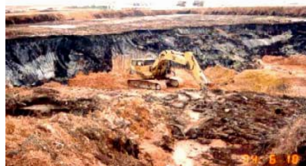
Fig. 1 Excavation and replacement of unsuitable materials
