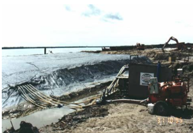
Fig. 12 Vacuum consolidation for the New Kuching Deepwater Port at Kg. Senari, Sarawak
