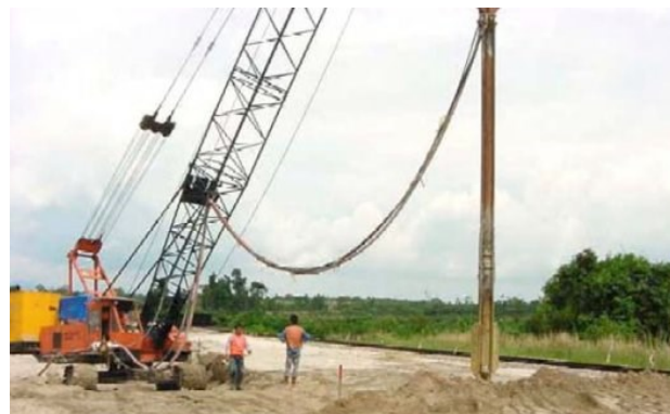
Fig. 19 Electric vibroflot for sand compaction
