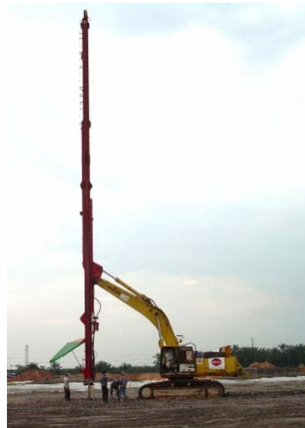
Fig. 8 Installation of vertical drains using hydraulic rig.
