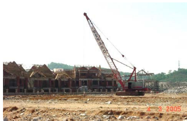
Fig. 15 Dynamic compaction at Bandar Menjalara for double storey houses on non-engineered filled ground.
