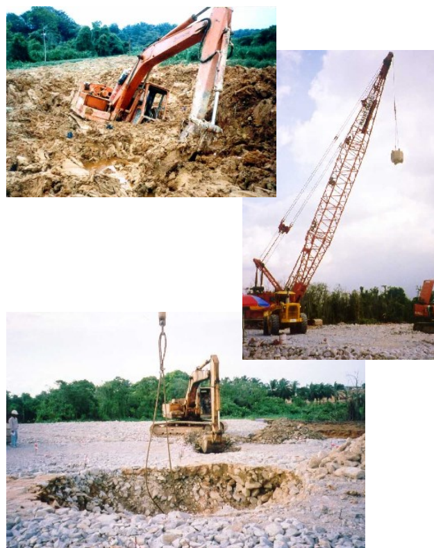
Fig. 28 Site condition before treatment (top); 300 ton.m DR rig (middle) and 3.5m diameter DR rock column (bottom) at Senai.
