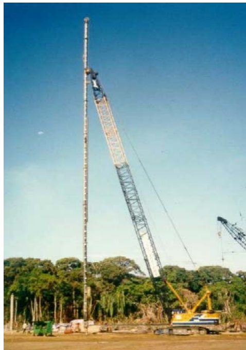
Fig. 7 A 50m-vertical drain installation at Miri
