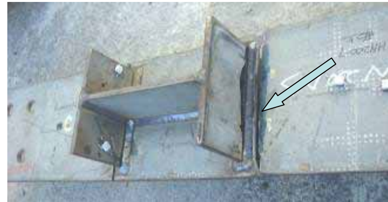
Fillet welded ribs
