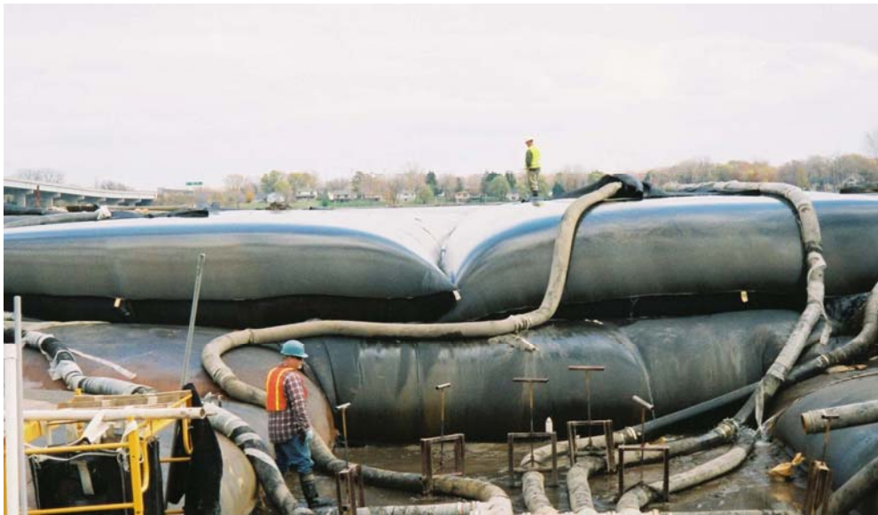
Geotextile tube inlet feeds
