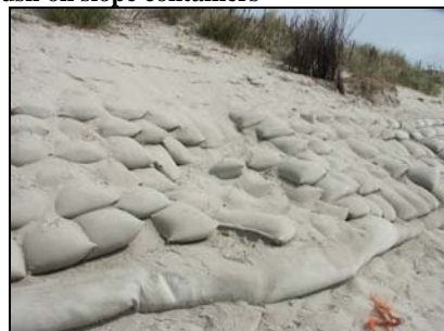
c) Pull out effect in a dune reinforcement (Courtesy by Heerten)
