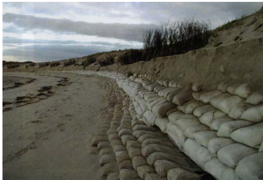
c) Dune Reinforcement in Wangerooge, North Sea/Germany (Vohlken et al, 2003)
