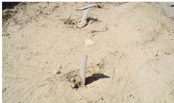
Figure 1-2. Supplementary Pre-installed Wick Drains
