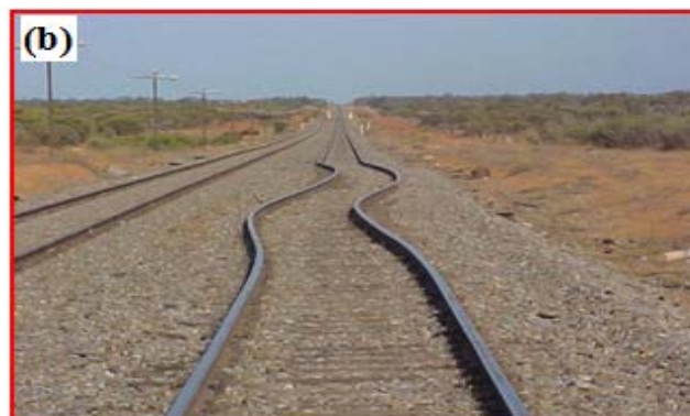
Figure 1 (a) Ballast breakage in a rail track (b) Buckling of track due to insufficient lateral confinement (After Indraratna et al. 2011); (Quoted by Syed Khaja Karimullah Hussaini, Buddhima Indraratna, and J. S. Vinod, 2018)
