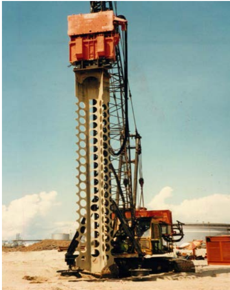
Application of Deep Vertical Vibratory Compaction Using Resonance Amplification, after Massarsch (2023)
