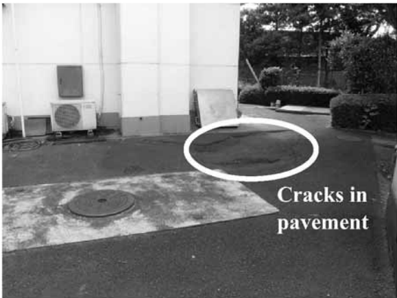
Fig. 9.41 Differential settlement around building
