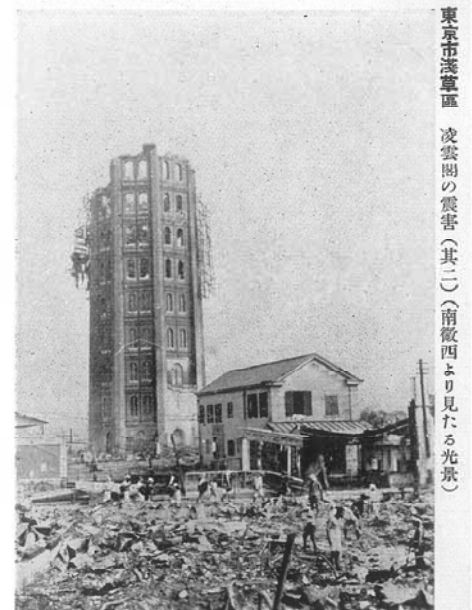
Fig. 7.1 Destroyed tower in Tokyo during 1923 Kanto earthquake (photograph from JSCE report)
