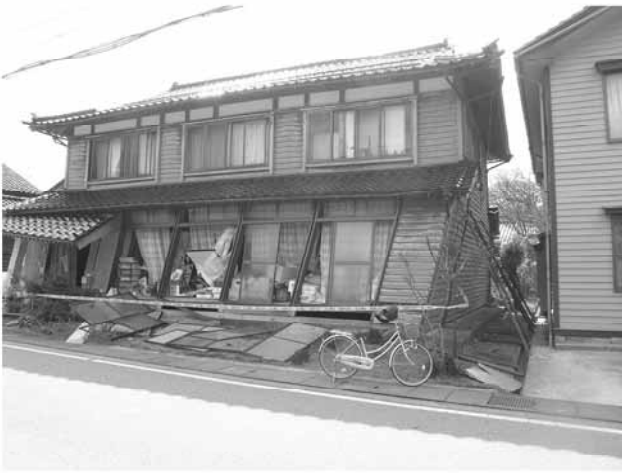
Fig. 5.41 Tilting towards direction of no wall rigidity Fig. 5.42 Dislocation of house from foundation
