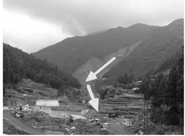
Fig. 15.59 Motion of mass along slope surface Fig. 15.60 Changed flow direction of debris at bottom of slope (rainfall-induced slope failure in Shikoku, Japan, in 2004)
