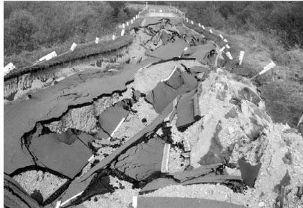
Fig. 14.12 Failure of road embankment at Chiebunnai Bridge in 1994
