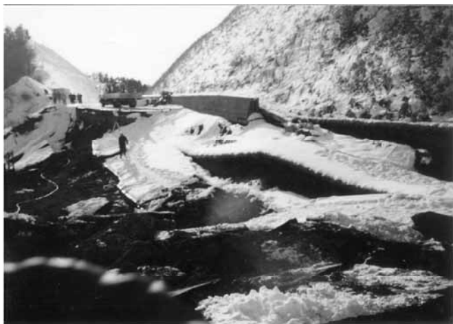
Fig. 14.43 Failed shape of Itoizawa road embankment in 1993
