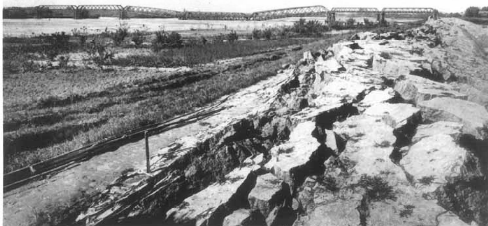
Fig. 14.14 Cracks at the top of Nagara River dike caused by 1891 Nobi earthquake (Photo supplied by Ministry of Construciton)
