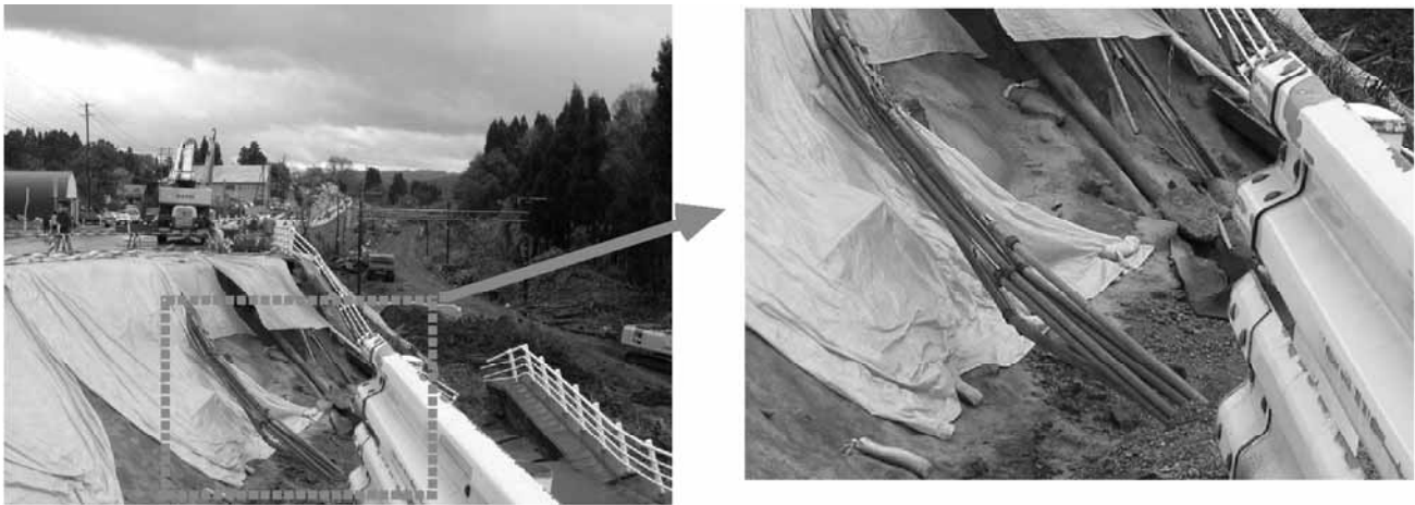
Fig. 14.4 Effects of collapse of road embankment on embedded lifelines
