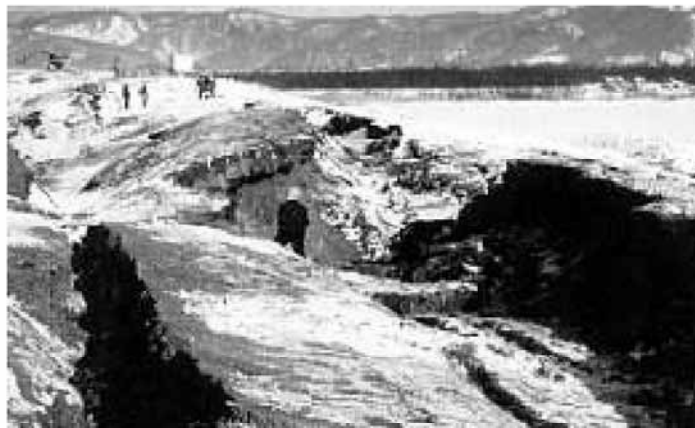
Fig. 14.11 Slump failure of road embankment due to subsoil liquefaction (Akita Sakigake Newspaper)
