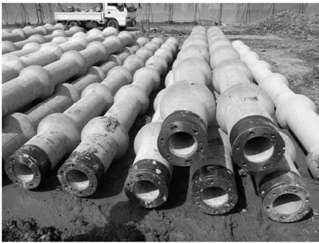
Fig. 13.31 Nodular piles prior to installation
