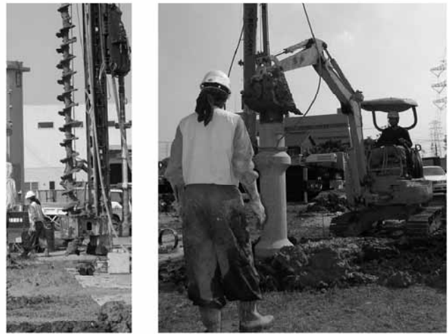
Fig. 13.32 Installation of nodular pile
