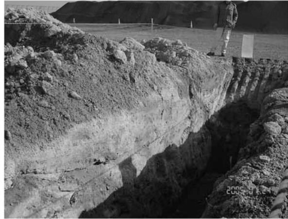
Fig. 10.71 Trench cut in landfill of incinerated ash in Tokyo
