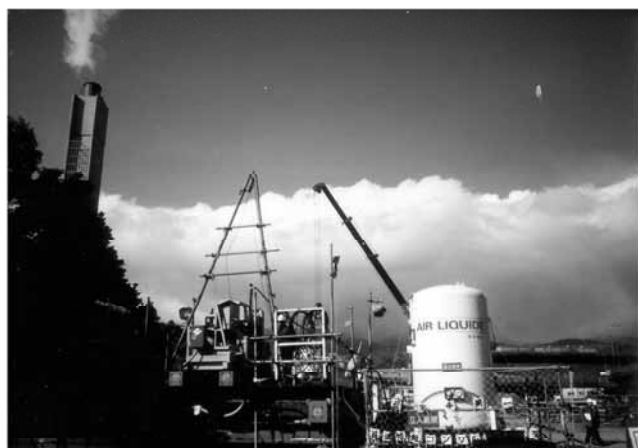
Fig. 10.63 Practice of in-situ freezing (in Uozaki)
