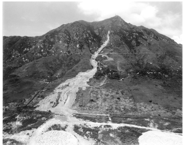
Fig. 25 Debris flow at Tsing Shan in 1990
