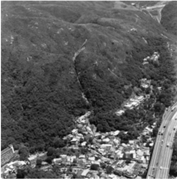
Fig. 27 Debris flow at Sham Tseng San Tsuen in 1999
