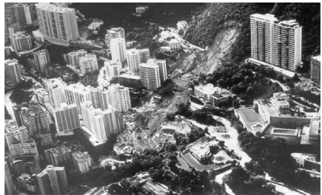
Fig. 2 1972 Po Shan Road Landslide
