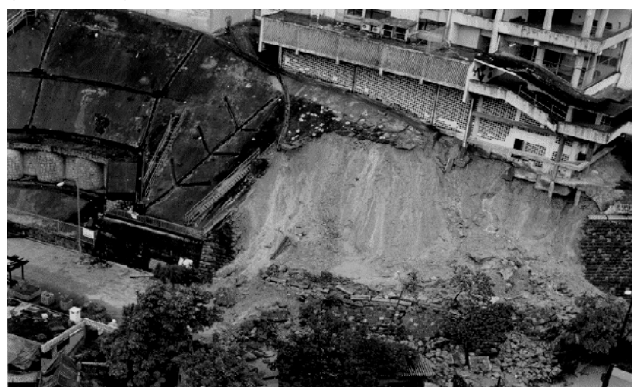
Fig. 11 1994 Kwun Lung Lau landslide
