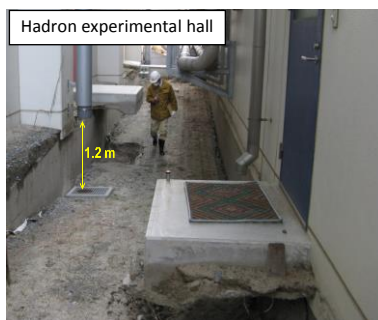
(a) Ground subsidence along building
