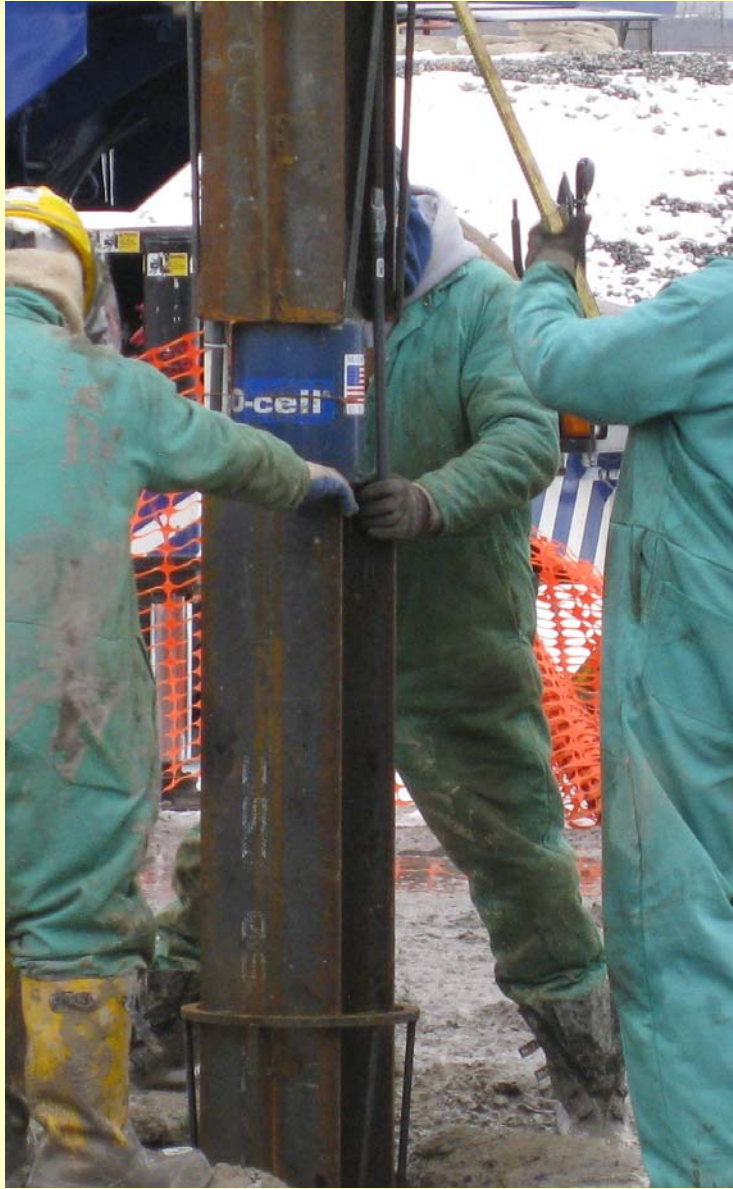
O-cell in a pipe pile inserted in a augercast pile after grouting.
