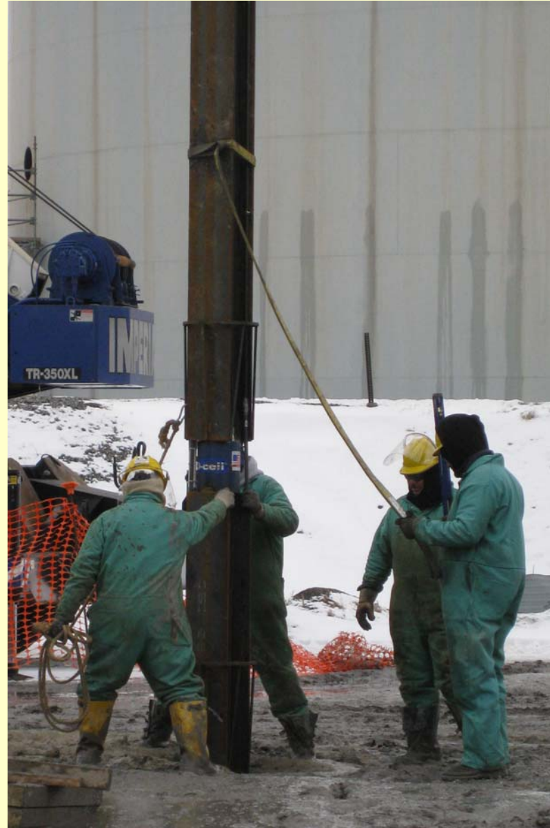
O-cell in a pipe pile inserted in a augercast pile after grouting.
