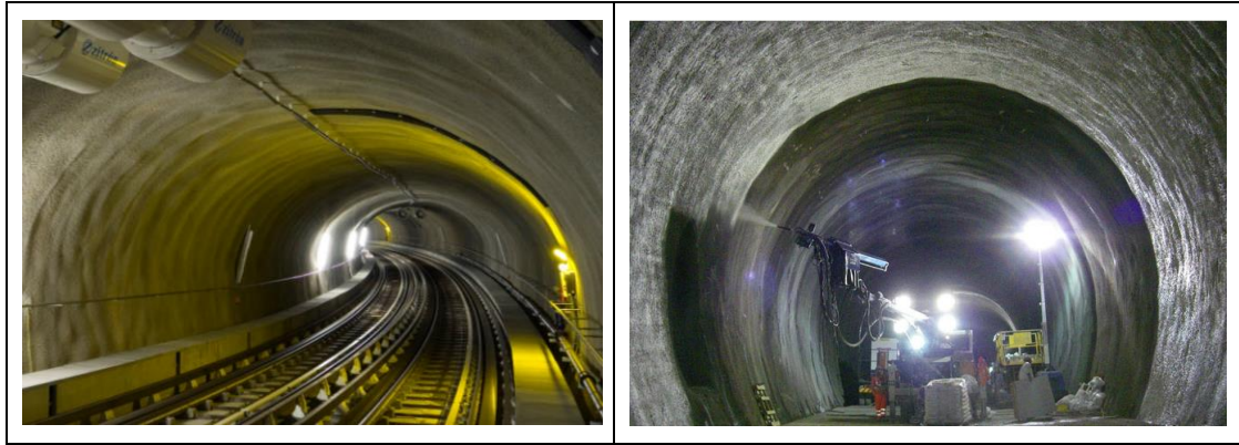
Figure 4 Two tunnels where single-shell construction with sprayed-membrane for water control has been the successful solution. The tunnel on the left is from the Lausanne metro (photo: Karl Gunnar Holter), and the tunnel on the right is the Hindhead main road tunnel in England during final shotcreting. (Photo:Shani Wallace, Tunnel Talk, July 2011).
