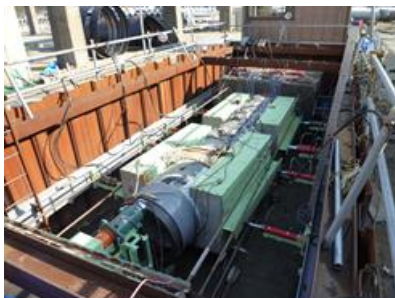
Pipe Jacking (after Le et. al, 2013)
