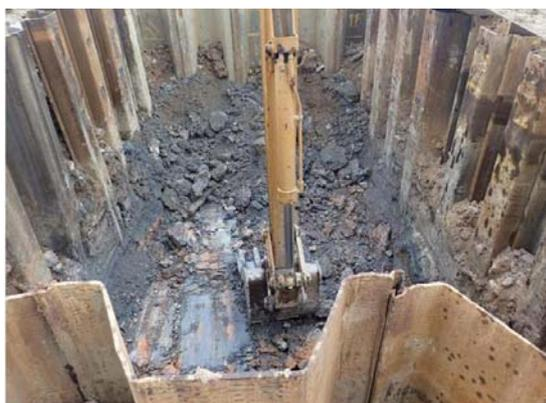
Figure 31 Cofferdam excavation
