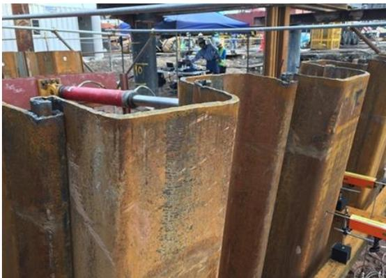
Figure 8 Interlock slippage at the top portion of the IV-pile wall
