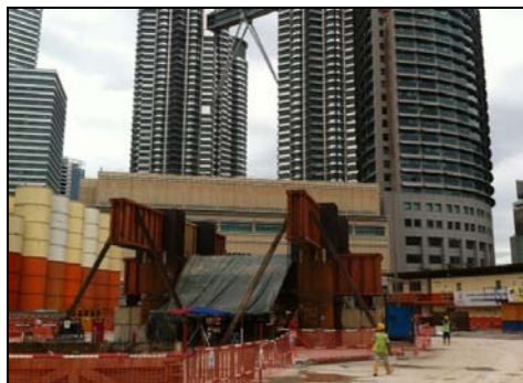
Figure 3 Reaction Pile Load Test
