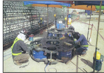
Figure 4 Bi-directional Load Test
