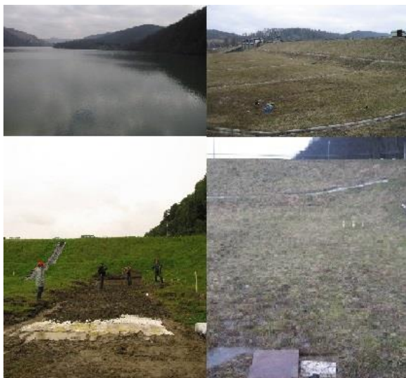
Figure 8 Installation of a GOF-based non-woven mat behind an earth dam in Myczkowce, Poland
