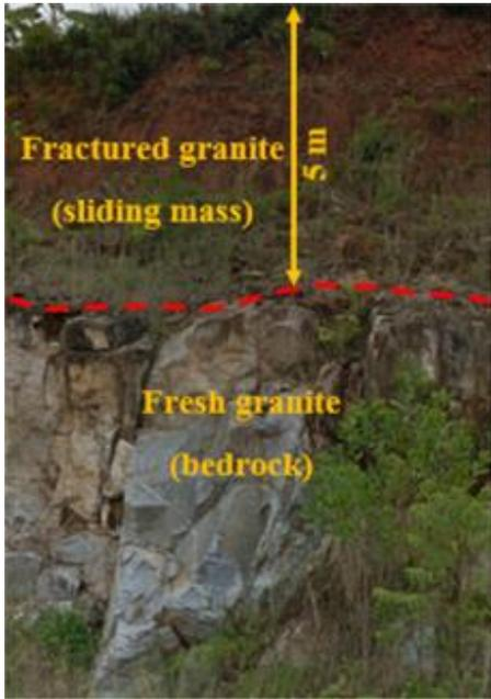
Figure 2 Exposed Geological Section in the study area
