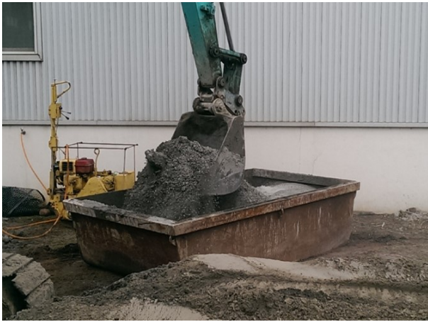
Figure 5 On-site mixing of pervious-CLSM with the bucket of a backhoe
