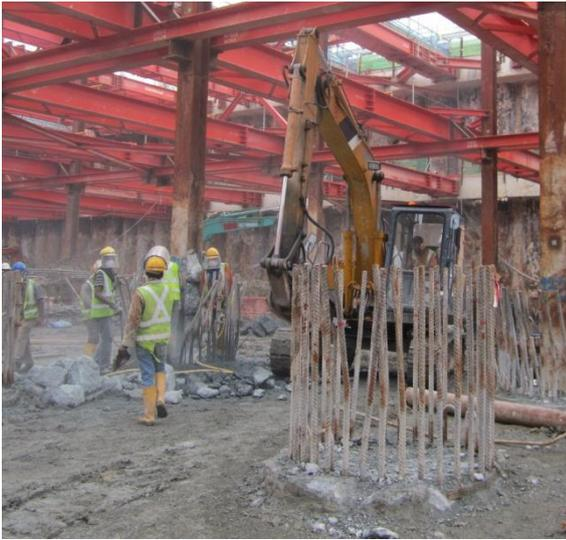
Figure 1 Deep excavation in Singapore with exposed ground improvement
