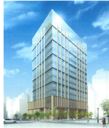
Figure 15 Exterior (building B)
