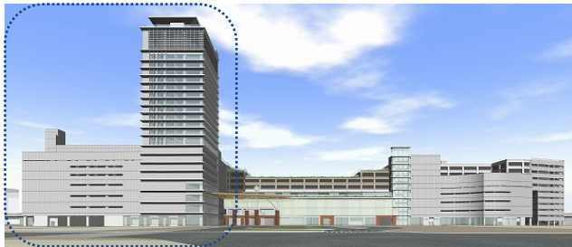
Figure 2 Exterior (building A)
