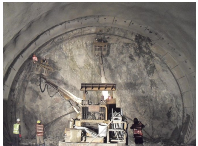
Figure 40 Steel rib (Lattice girder) installations
