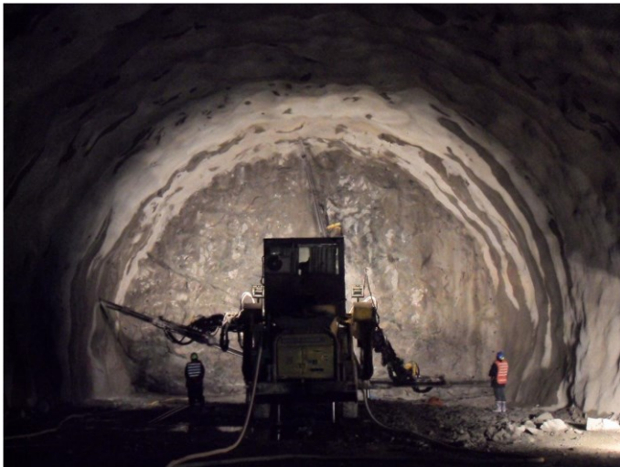
Figure 37 Drilling works for the blasting
