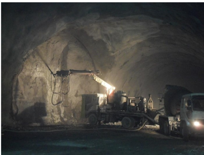
Figure 38 Shotcrete placements after the blasting
