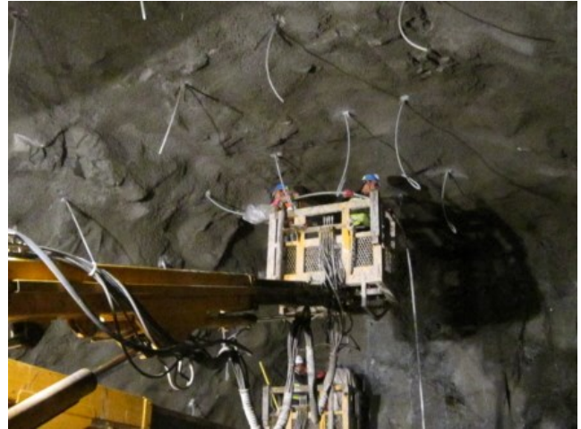
Figure 39 Rock bolt installations
