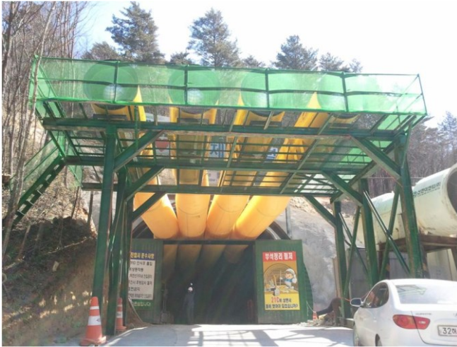
Figure 36 Ventilation tubes for construction (110 KW)
