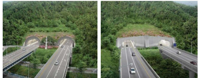
Figure 25 Portals at both ends of the tunnel
