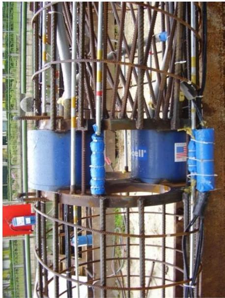
Figure 13 Reinforcement cage welded onto bearing plates of BD-cell (Courtesy of Foundation Alliance, 2018)
