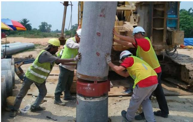
Figure 14 Installation of BD-cell in precast pile (Courtesy of YJack, 2018)
