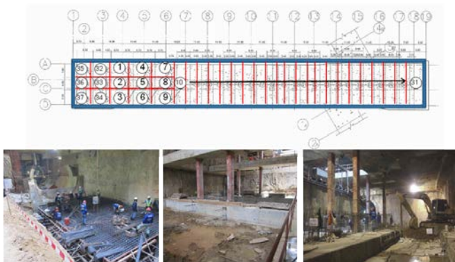
Fig. 10 Sequence of staged base excavation of BS13
