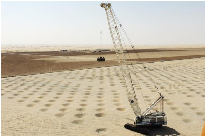
Figure 12 Dynamic compaction rig and impact craters
