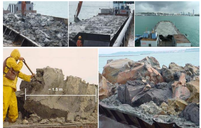
Figure 3 Transportation of dredged materials by barges (top) and dredged clay lumps (bottom)
