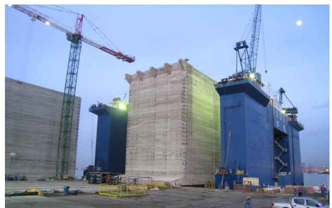
Figure 8 Completed caissons at the fabrication yard
