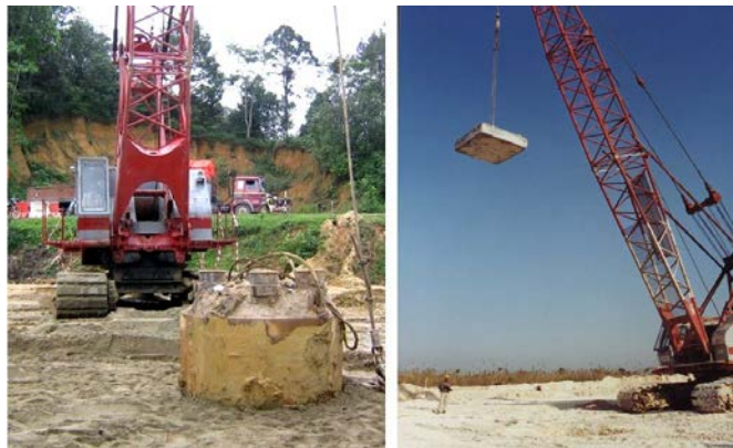
Figure 16 Punching DR pounder (left) and flat DC compaction pounder (right)
