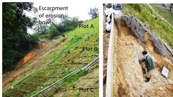
Figure 3 Slope failure and its escarpment at Plot A
