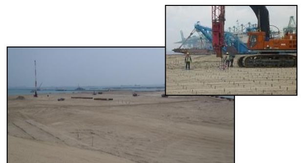
Photo 3 Reclamation of sand fill and PVD installation
