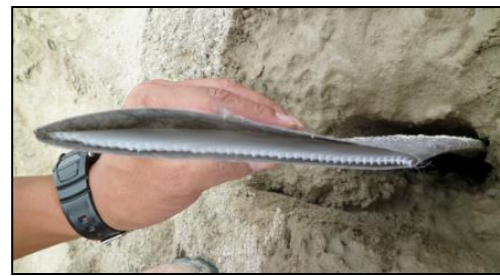
Photo 4 Installed prefabricated vertical drain
