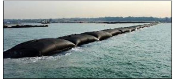
Photo 11 Containment bund completed by geotextile tubes and infill of CMS
