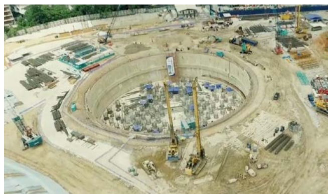
Circular cofferdam with 76m diameter
