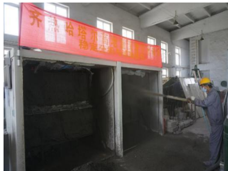
(b) Spraying concrete
