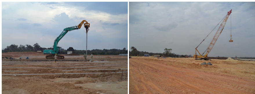
Figure 12 Site construction photo
