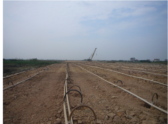
Figure 2 Array of vacuum pipes and horizontal drainage pipes
