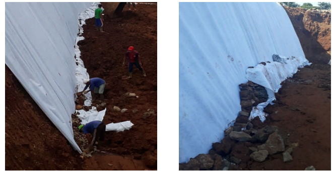
Figure 9 Installation of Gravel as a Drainage Material
