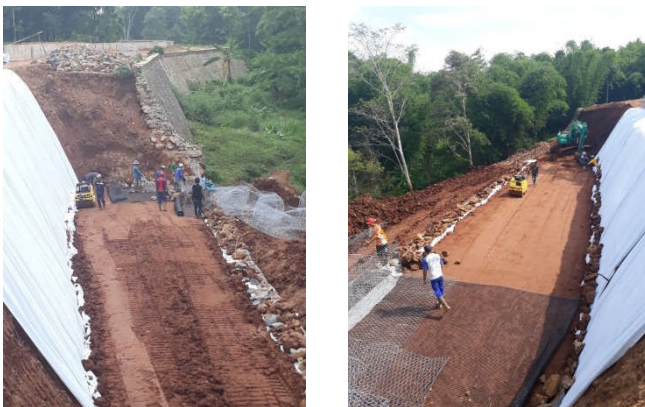
Figure 8 Installation of Terramesh and MacGrid as Reinforced Soil Structure
