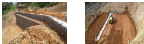
Figure 15 Backfill and Compaction Procedures
