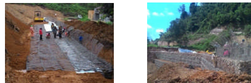
Figure 14 Paralink Installation (Left) and Terramesh Installation (Right)
