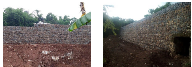
Figure 10 View of the Reinforced Soil Structure during construction (left) and almost completed (right)
