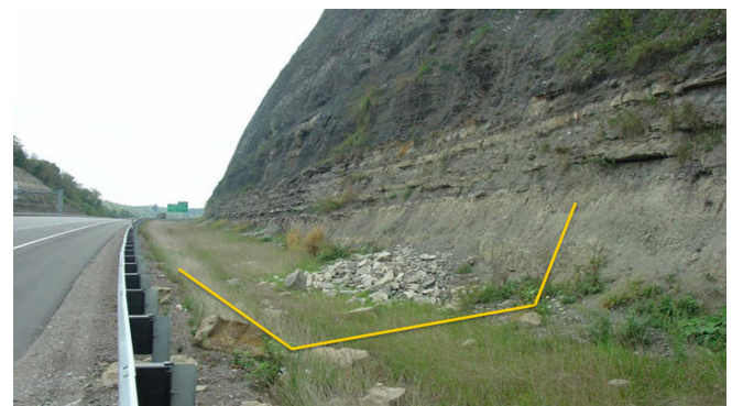
Figure 3. Example of a simple drapery mesh with a ditch (highlighted with the yellow line) at the base to collect the debris falling from the slope
