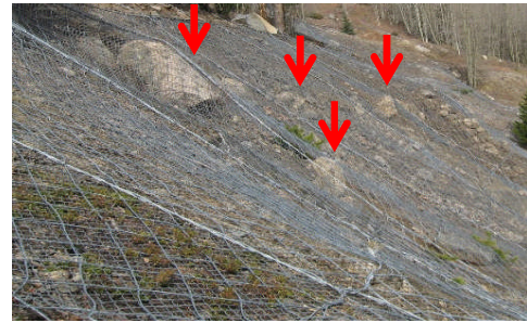
Figure 8. Example of a simple drapery system with cable panels and double twist mesh. The proper weight of the meshes (approx. 5.0 kg/m 2 ) can avoid the rolling of single boulders (red arrows) along the slope.
