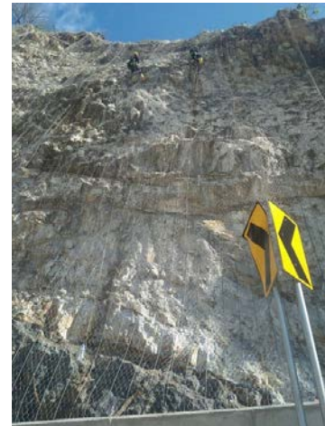
Figure 19. Installation of rockfall netting for Maros elevated road.
