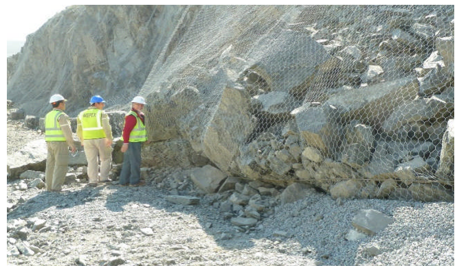
Figure 2. Debris and rock piled up at the bottom of a simple drapery system fixed at the toe of the slope by anchors and a down-slope longitudinal cable
