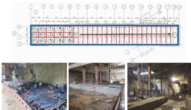
Fig. 10 Sequence of staged base excavation of BS13
