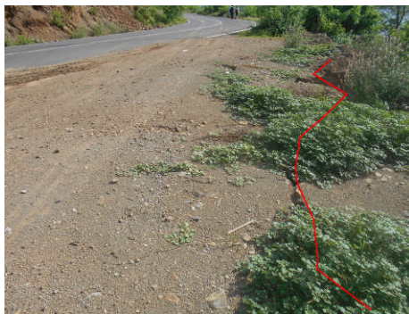
Figure 2: Initial crack above the site project
