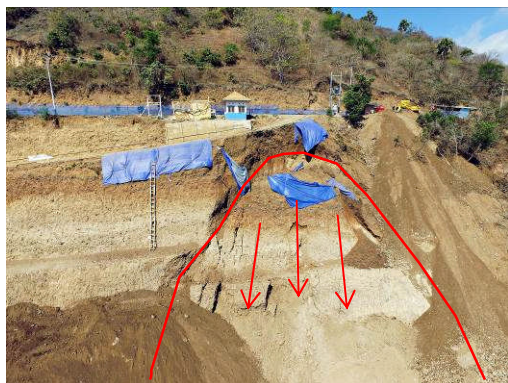
Figure 3: Post-Slope failure Condition.
