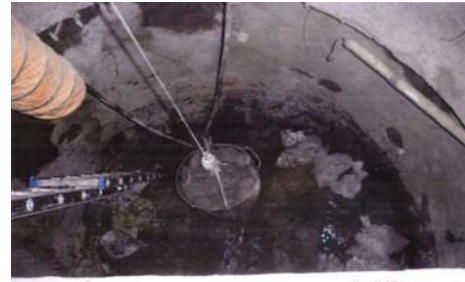
Figure 6 Muddy water started to flow into the bottom of the sump (4:15pm, December 4th, 2005)
