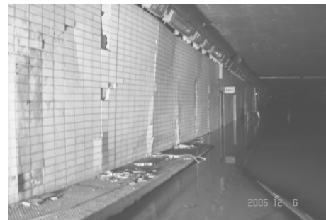
Figure 13 the sinkhole development on the north side above the down track tunnel (4:30pm, December 5th, 2005)
