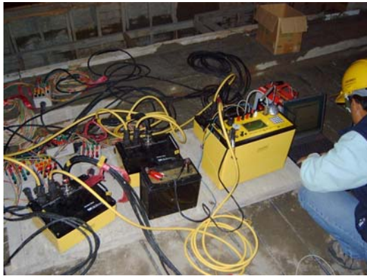
Figure 18 RIP Testing equipment
